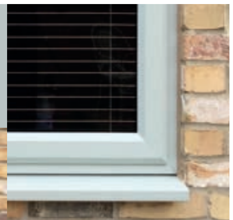
Welded joints on both outer frame and Rebated Sash
