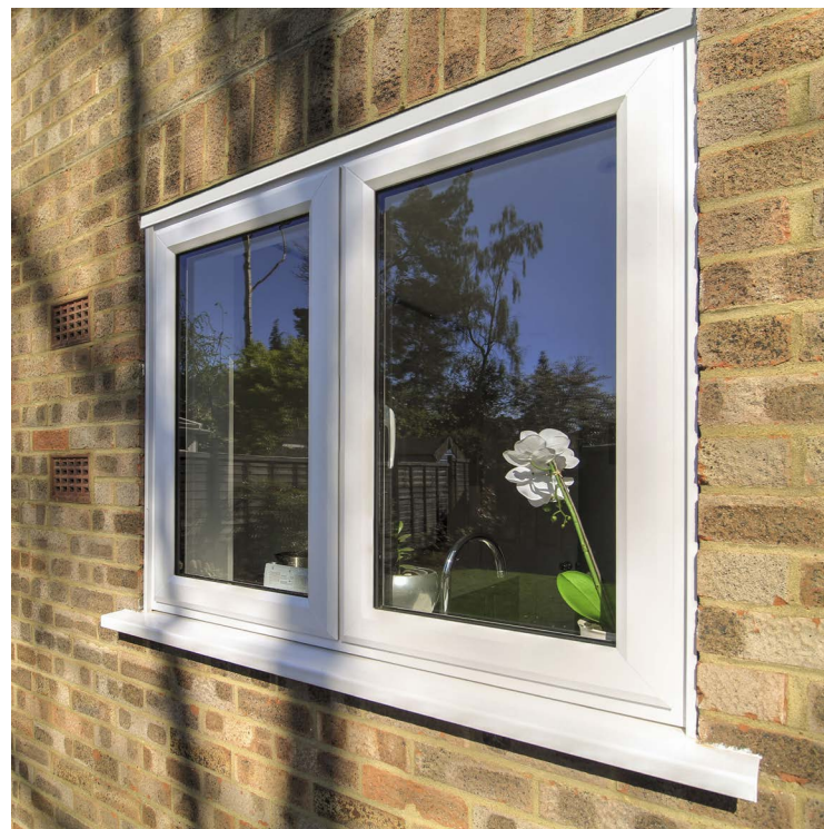
Concealed Ventilation installed through the outer frame
